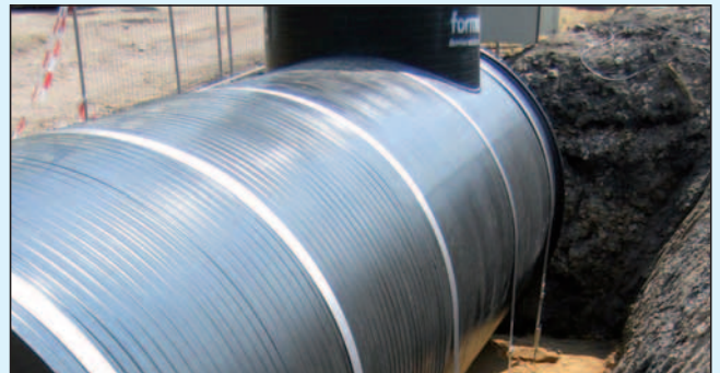
Stainless steel belts secure against buoyant uplift
