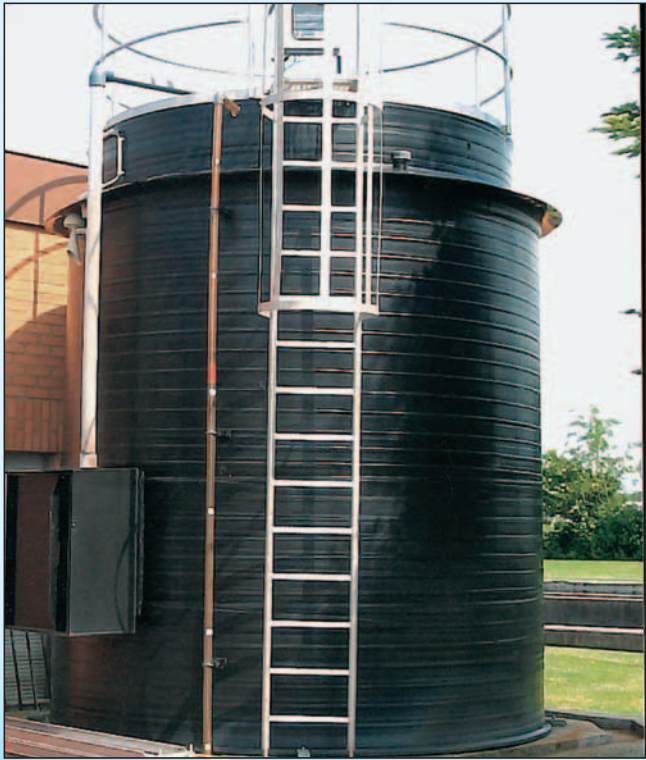
formoplast storage tank with secondary containment shell. Contents: coagulant from water treatment plant. Capacity: 25,000 L, diameter: 3000 mm, overall height: 4700 mm
