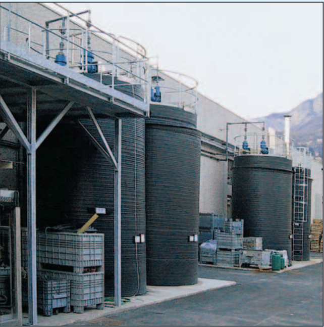
formoplast helically wound HDPE storage tanks with secondary containment shells, for storage of 50% sodium hydroxide, 50 % nitric acid and 96 % sulfuric acid. Capacity 30,000 L, diameter 2800 mm, height 5280 mm.
