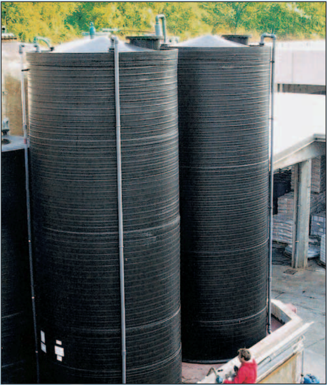
formoplast helically wound HDPE storage tanks, installed in owner's concrete catchment basin. Contents: 75 % phosphoric acid. Capacity: 50,000 L, diameter: 3000 mm, height: 7500 mm
