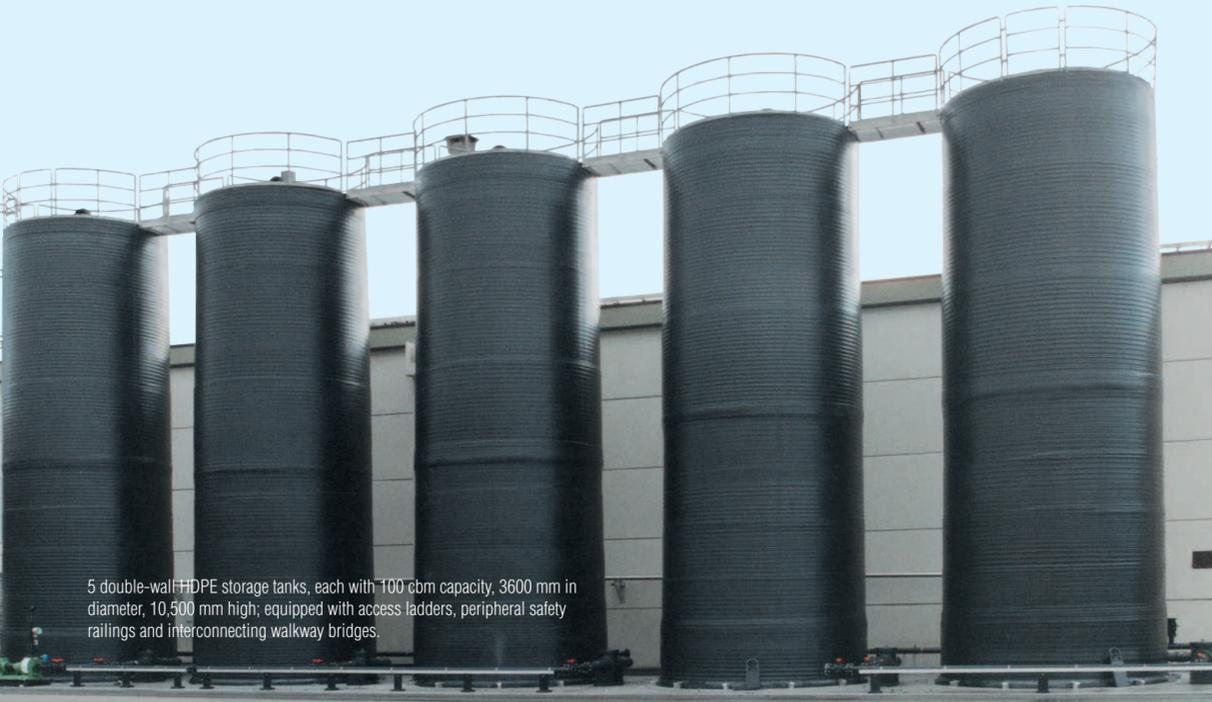
5 double-wall HDPE storage tanks, each with 100 cbm capacity, 3600 mm in diameter, 10.500 mm high; equipped with access ladders, peripheral safety railings and interconnecting walkway bridges.
