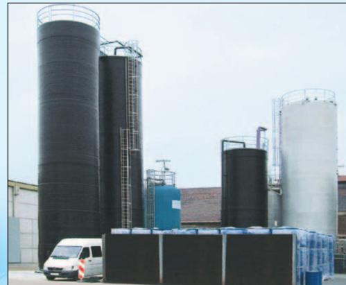
2 double-wall HDPE storage tanks, diameter 4000 mm, overall height 17,120 mm, capacity 200,000 L
